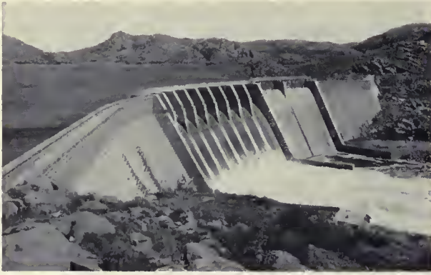
ALTUS DAM —one of the Bureau of Reclamation projects which supplies municipal water. Photo by P. W. George, Region 5.
